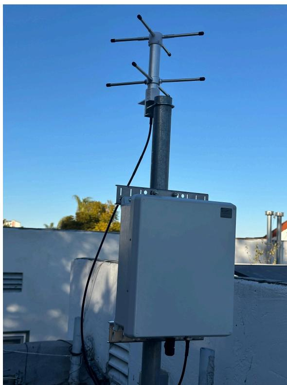
Some suitable antenna types for a fixed mount are eggbeaters, quadrifilar helices (QFH), or turnstiles (aka “crossed dipoles”). These all offer circular polarization, mostly omnidirectional radiation patterns, easy mounting, and insensitivity to nearby ground planes. Between each other, they vary a small amount in performance and mounting specifics.
